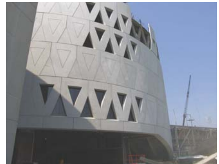
Figure 10: Construction photo of north side of building.
